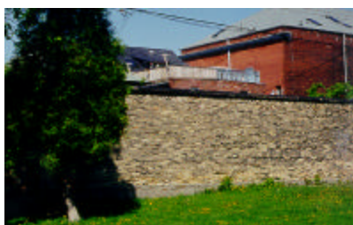
Top: The south wall, with portions missing; historic brick storage building.
