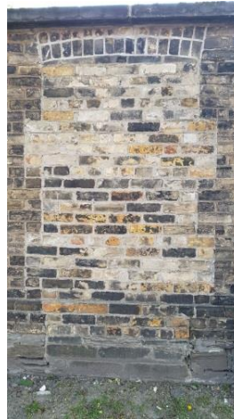
Figure 11: Bricked-in doorway in Bay 32.
