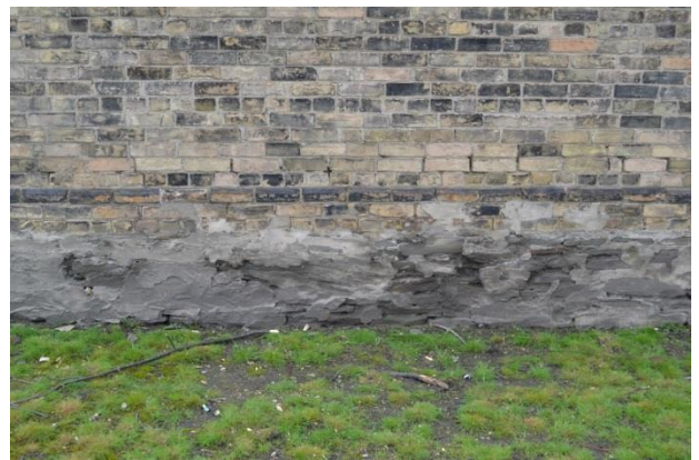
Figure 42: Stone foundations are recommended for rehabilitation.
