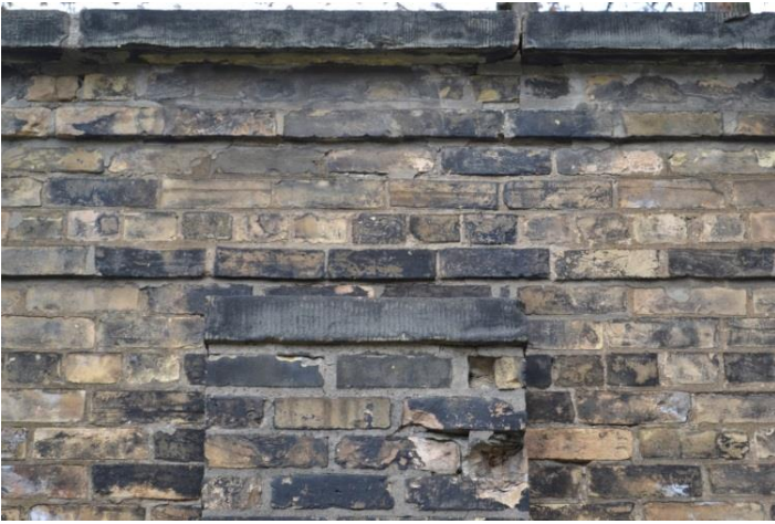
Figure 12: Brick corbels on higher portion of the wall.
