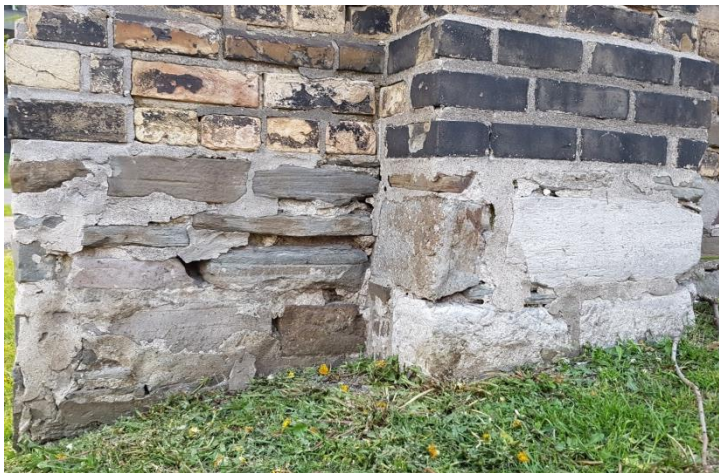
Figure 5: Typical ashlar stone pier and rubble wall foundations on east elevation.
