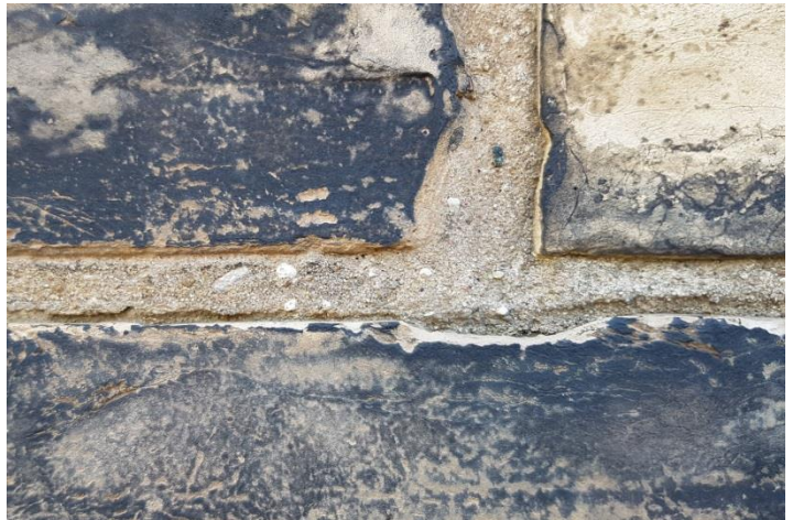
Figure 15: Close-up of mortar.
