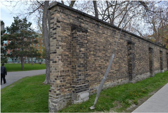
Figure 2: General view of the east elevation – Segment 10.
