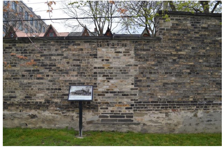
Figure 13: Exposed rough masonry foundations and raised sill of doorway.
