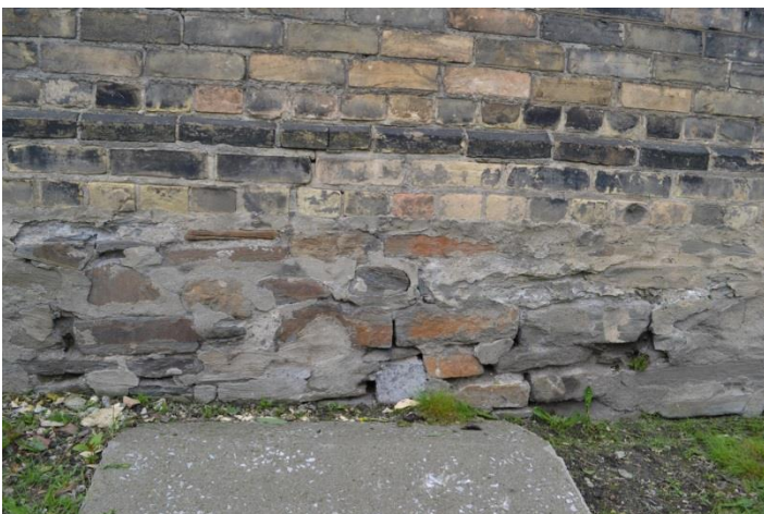
Figure 6: Typical rubble stone wall foundations on west elevation.
