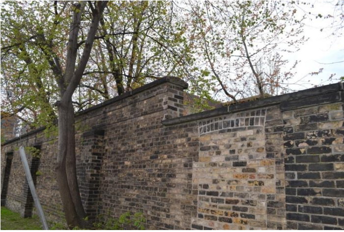
Figure 8: General view of east elevation showing change in height at Bay 32.
