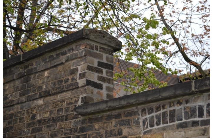
Figure 9: Close-up of end wall showing Lewis hole and newer bricks.
